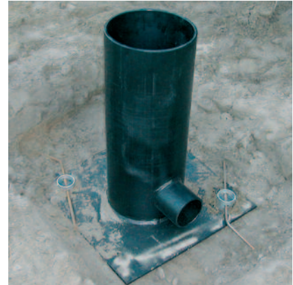
The foot support, a PE construction, anchored to the ground.
