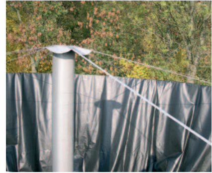
Specially constructed top end of the pole with seams.
